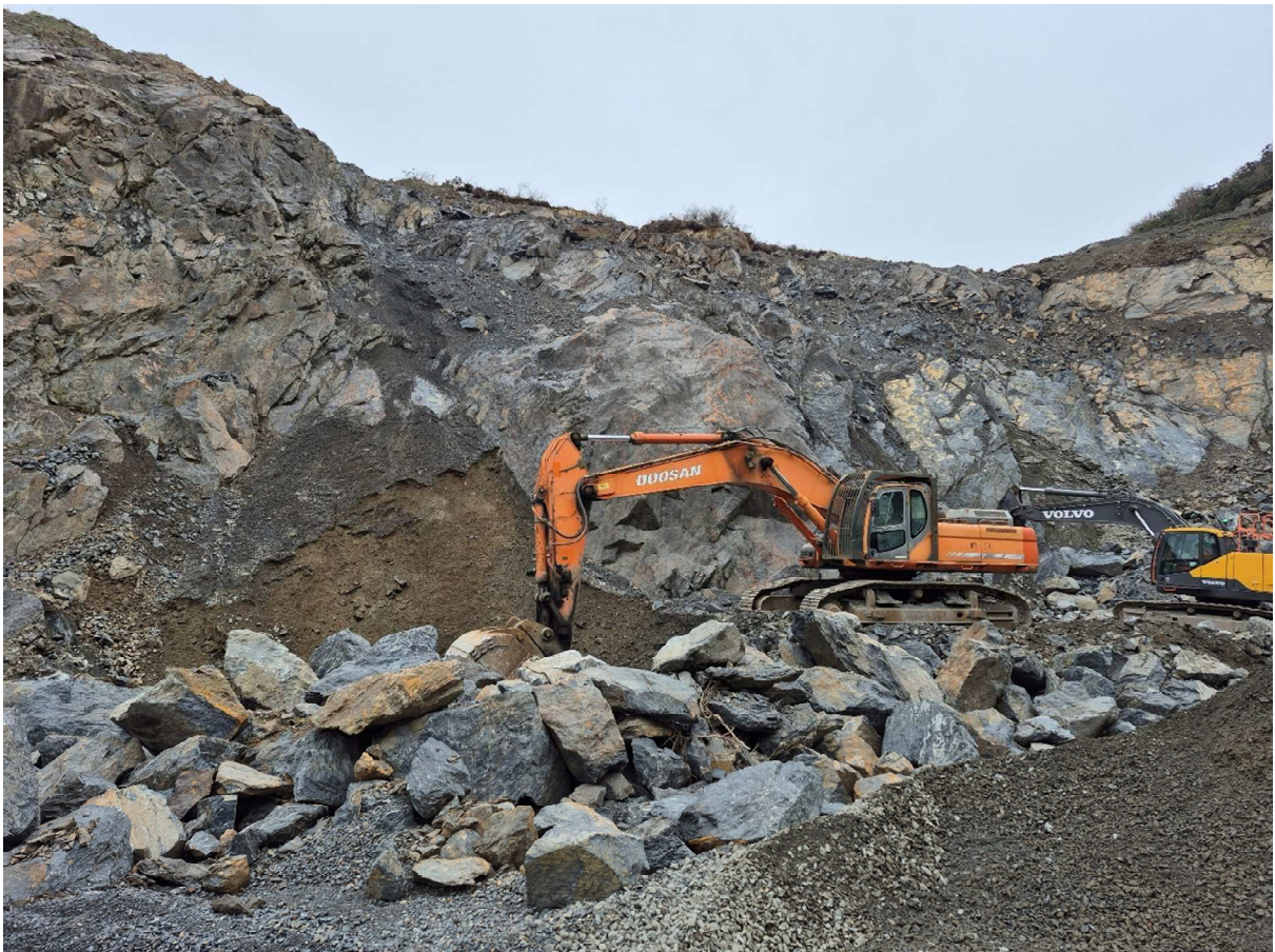
FIGURE 5: PLANNED DEVELOPMENT – NORTHERN FACE OF LOWER BENCH (LOOKING NORTH)
