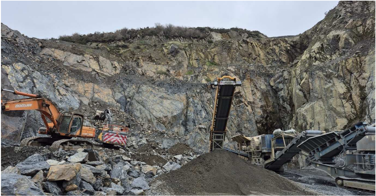
FIGURE 4: CURRENT DEVELOPMENT (LOWER BENCH, LOOKING EAST)
